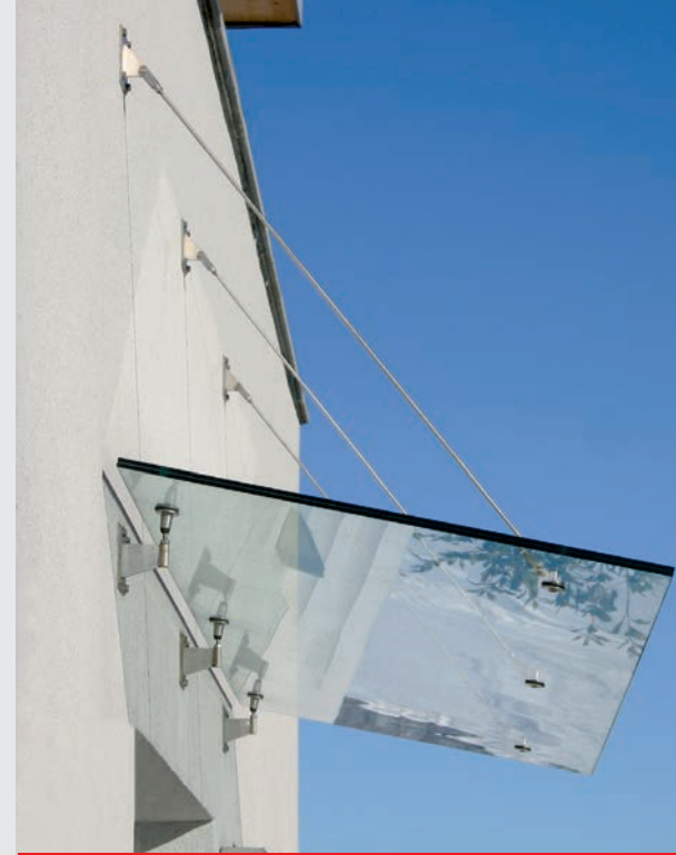
Glass holding system for canopies made of glass
